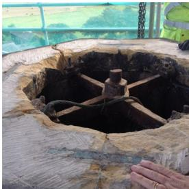
The picture is of the existing cast iron 'cross tree' which is to be replaced with stainless steel. This steelwork supports the 'holding down' rod which keeps the spire under compression. Amazing!
